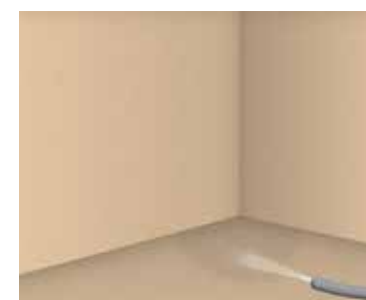
11 Fully broadcast the fresh primer with quartz sand
