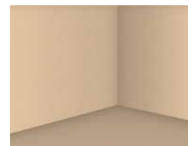
12 Completed walls and floor
